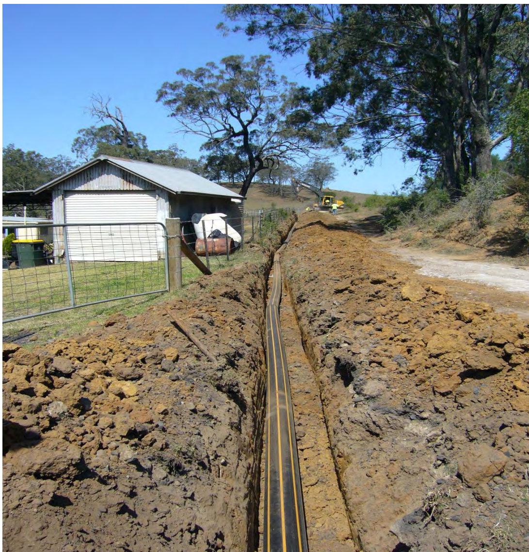
Illustration of a typical polyethylene gas gathering line being installed below the surface of a road verge at the Camden Gas Project
