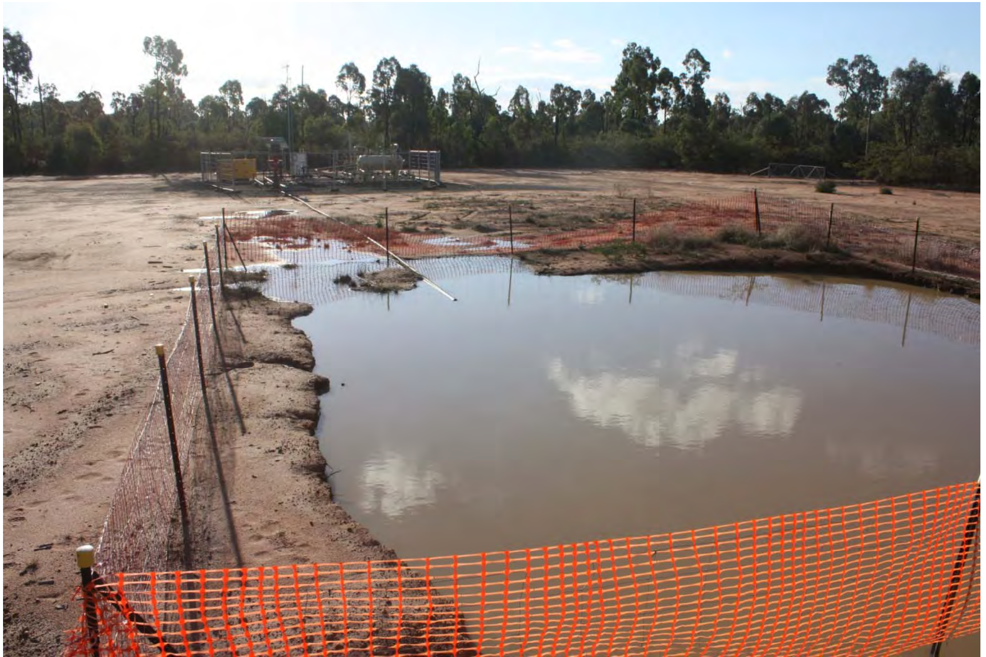
Overflowing unlined CSG holding pond – photo: July 2012
